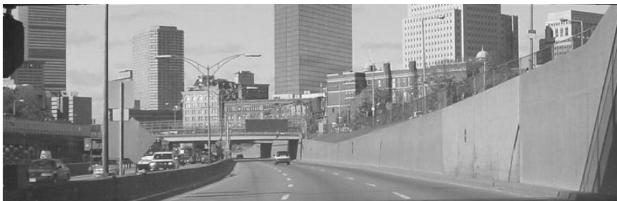
FIGURE A.3.3.36.1 Depressed Highway.
